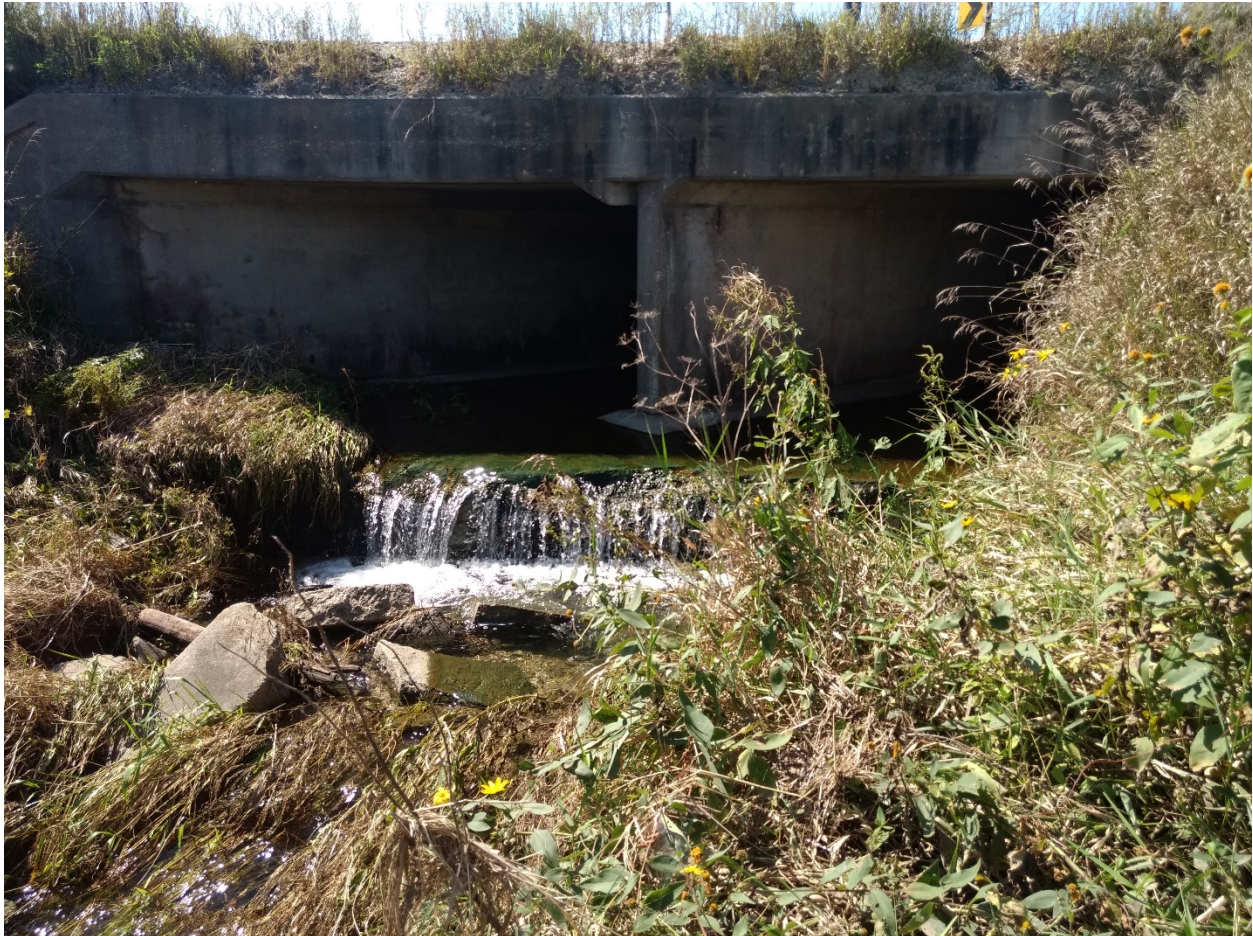
Twin Box Culverts, Mud Creek Tributary at 10 th Ave.
