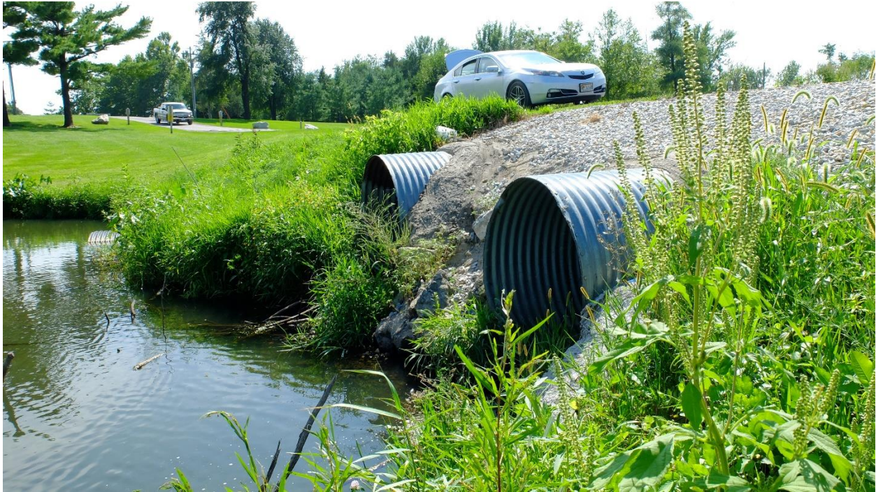
Twin culverts, main entrance road to Rodgers Park
